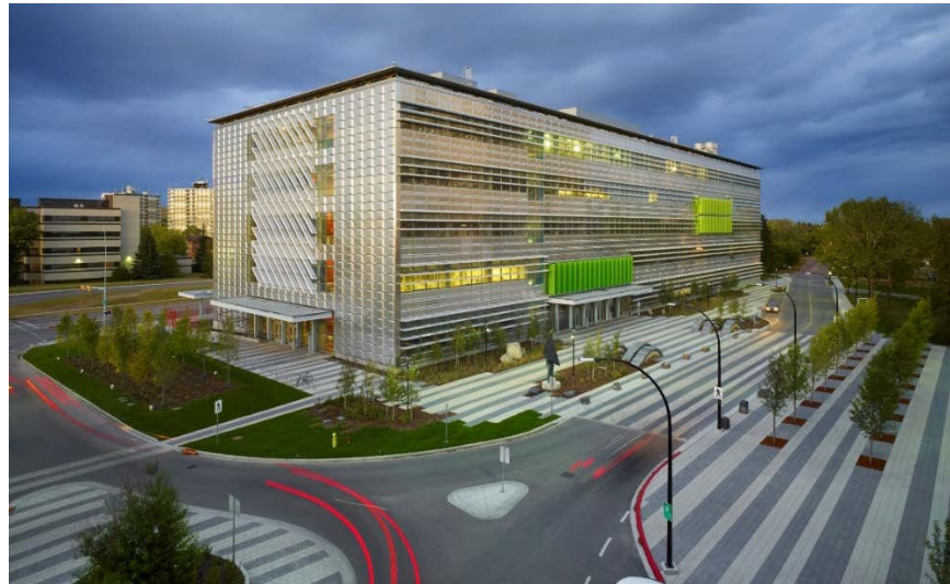
Figure 6. Energy Environment Experiential Learning Centre (EELC), University of Calgary. Source: https://www.archdaily.com/356805/energy-environment-experiential-learning-Perkins&Will (accessed on 5 July 2021). Reproduced with permission from Tom Arban Photography Inc.
