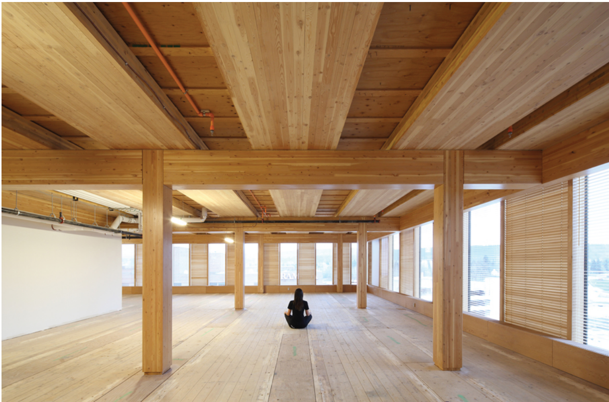
Figure 4. Wood Innovation and Design Centre by Michael Green Architecture. Photo: Ema Peter, 2015.
