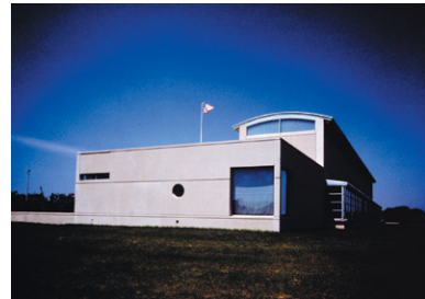
Fig.14 : View from parking lot. Spangler Semler Architects. Matteson Library Open Competition (1990-1992)
