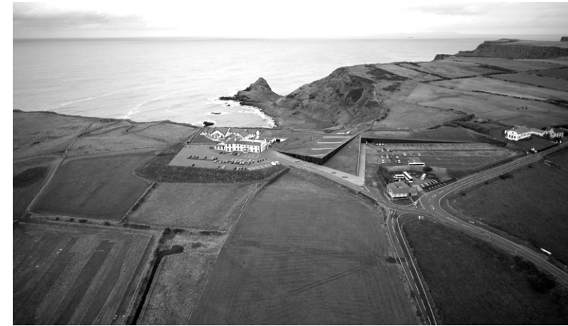
Fig.198 : Aerial view. Heneghan Peng Architects Dublin, Ireland Giant's Causeway Visitors Centre Antrim County, Northern Ireland Competition (2005) Completion (2012)
