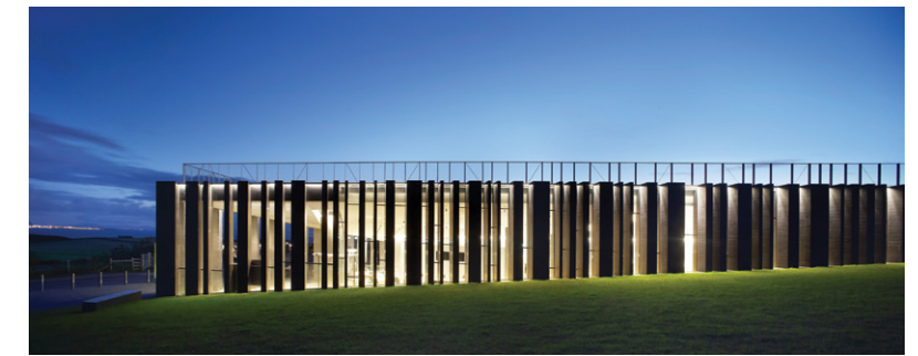
Fig.199 : Aerial view. Heneghan Peng Architects. Dublin, Ireland. Giant's Causeway Visitors Centre. Antrim County, Northern Ireland. Competition (2005). Completion (2012).
