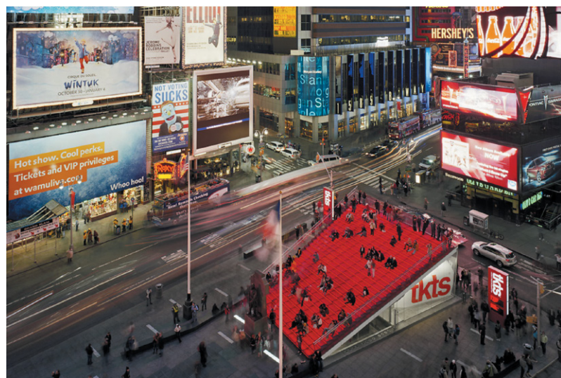
Fig.60 : Photo after construction of the glass enclosed structure. John Choi/Tai Ropiha. Times Square TKTs (2000). Perkins Eastman - Architects of Record.
