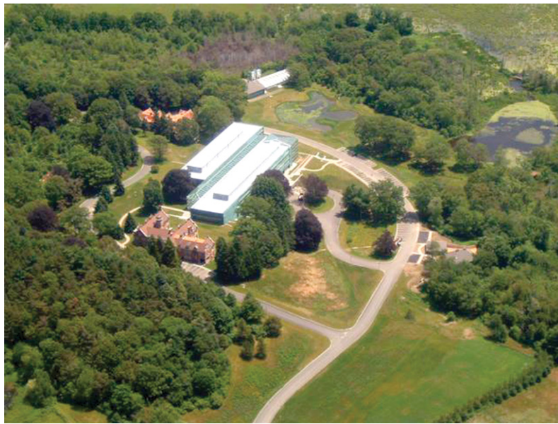
Fig.4 : Aerial view with waste water facility in background and estate house, used for company offices, in foreground. Weston Williamson . London, U.K./Melbourne, Australia.
