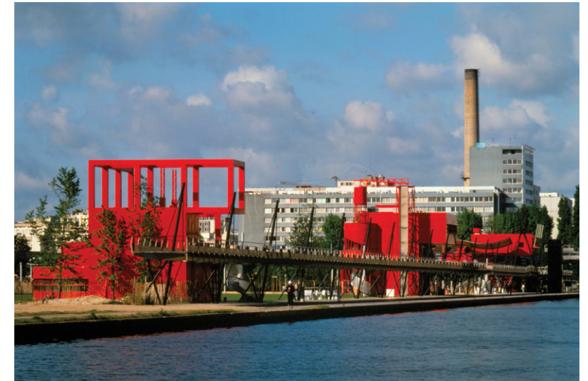
Fig.144 : Follies view. Parc de la Villette. Bernard Tschumi Architects. New York/Paris. Competition (1983). Completion (1987- )
