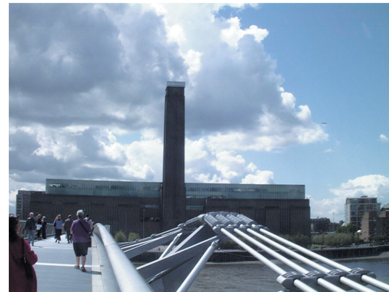
Fig.189 : View to Tate Modern Foster + Partners with ARUP. Millennium Bridge Competition (1996) London, U.K.
