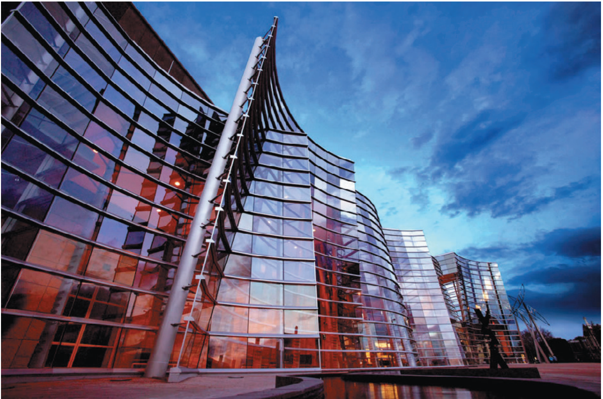
Fig.252 : Christchurch Art Gallery . Christchurch, New Zealand. Buchan Group . Sydney, Australia. Competition (1998). Completion (2003)
