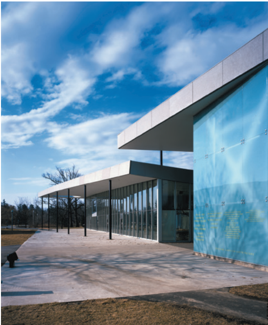
Fig.45 : South facade perspective. Kohn Shnier Architects . Toronto. University of Toronto. Mississauga Student Centre. Completion (1999)
