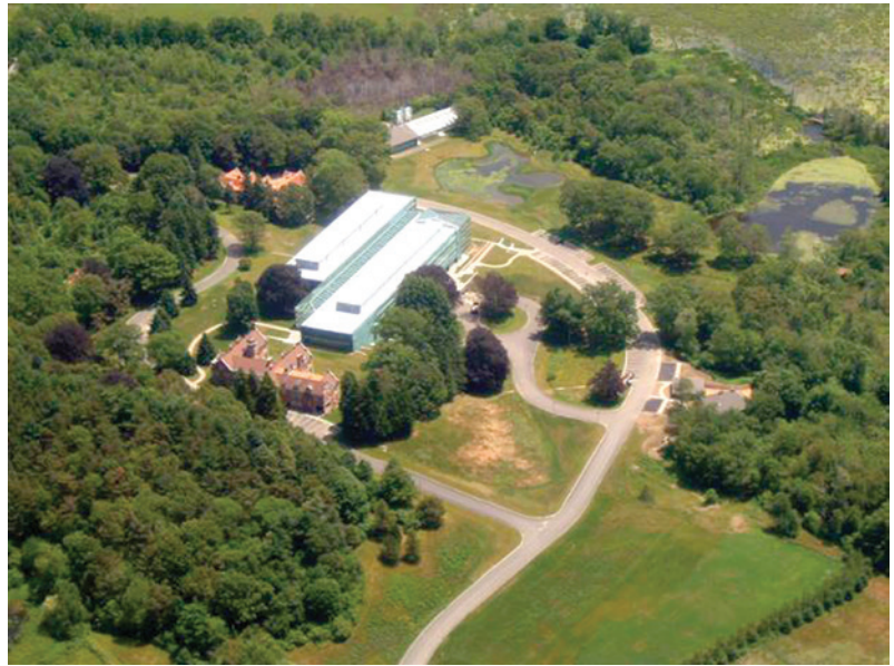
Fig.4 : Aerial view with waste water facility in background and estate house, used for company offices, in foreground. Weston Williamson . London, U.K./Melbourne, Australia.
