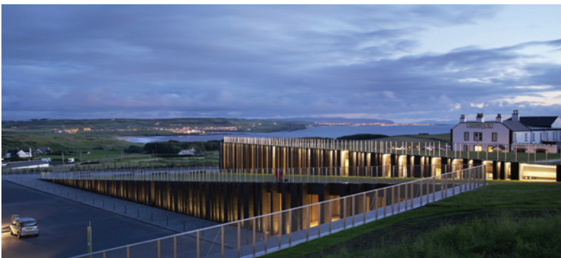
Fig.202 : Night View Heneghan Peng Architects Dublin, Ireland Giant's Causeway Visitors Centre Competition (2005) Completion (2012)
