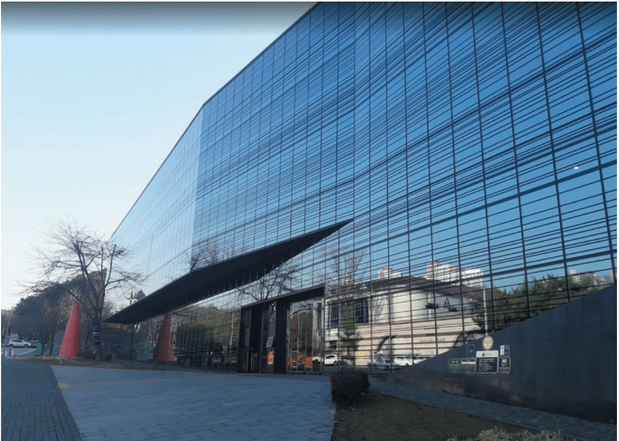
Fig.220 : Approach perspective. Nam June Paik Museum . KSMS Kirsten Schemel / Marina Stankovic Architekten BDA/ with Schlaich Bergerman Partner. Berlin/Stuttgart. Development Stage Architect : Marina Stankovic . Completion (2008)
